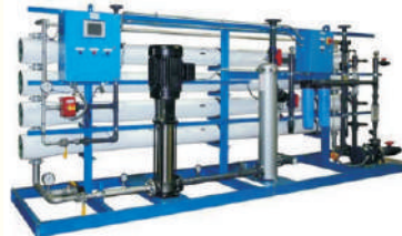
Building RO Plant
