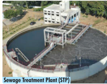
Sewage Treatment Plant (STP)
