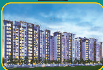
@ LOHEGAON Phase 3 Nearing Possession
