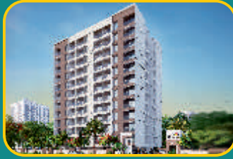
@ LOHEGAON Phase 2 Nearing Possession
