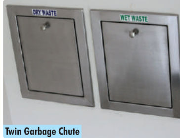
Twin Garbage Chute
