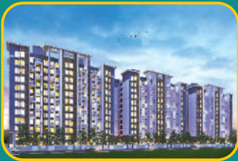
@ LOHEGAON Phase 3 Nearing Possession
