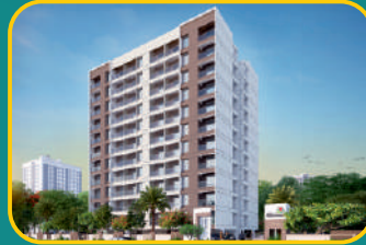
@ LOHEGAON Phase 2 Nearing Possession
